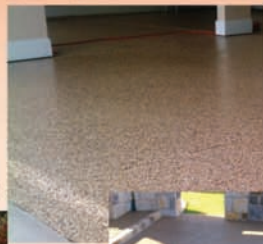
Garage floor Epoxy Chip Flake
