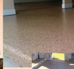
Garage floor Epoxy Chip Flake
