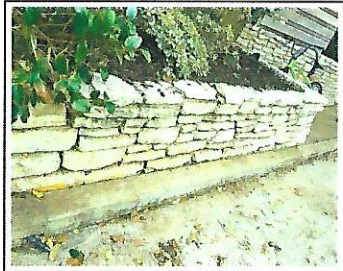
RAISED LIMESTONE PLANTER ROCK WALL
